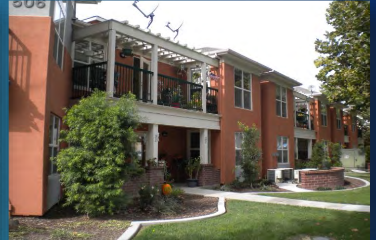
Town Center Senior Manor Corner of Plumas and B Street, Yuba City 28 units (senior housing)
