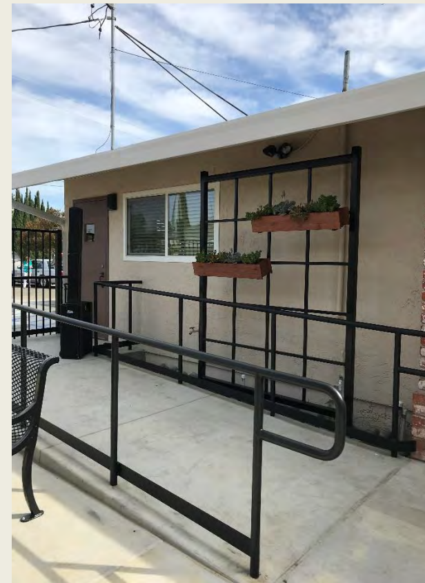
New ramps w/ railing
